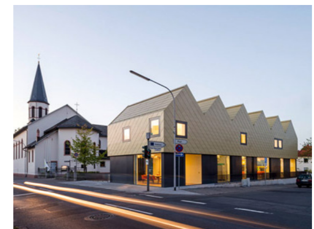
Community Centre in Urberach. Designed by Netzwerk Architekten
