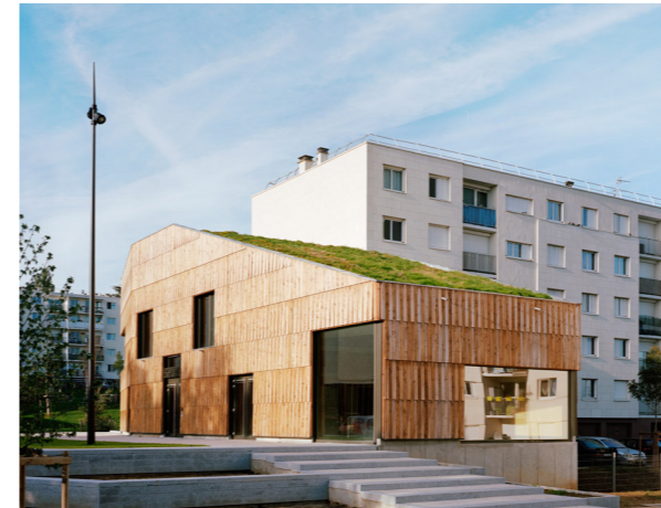
Centre Sociocultural. Designed by Guillaume Ramillien Architecture
